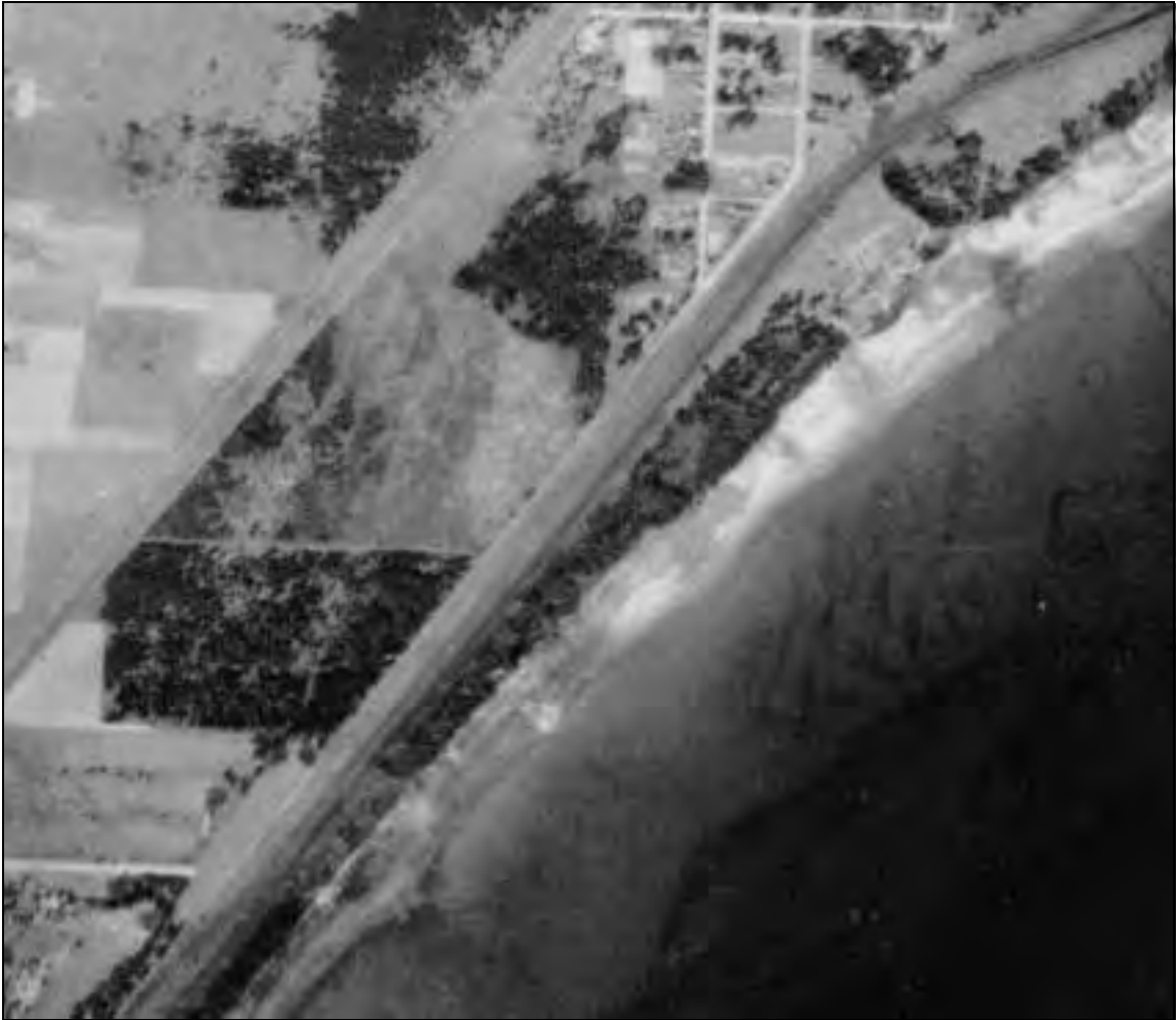
Plate 2. Black Rock Vicinity Aerial View, 1935.
