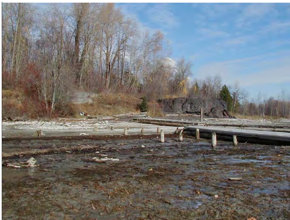
Figure 1. Overview of structural remains (left of center), slag (right of center), and dock pilings (foreground) of the Panhandle Smelter, direction: N.
