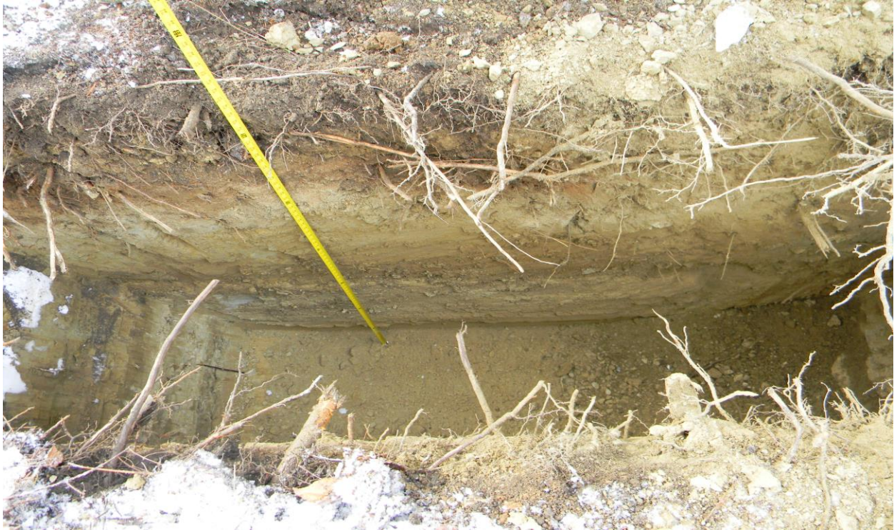
Figure 10. Photograph of TP 3 taken at the end of excavation. The exposed wall is 6 feet below the surface. The view is to the east.
