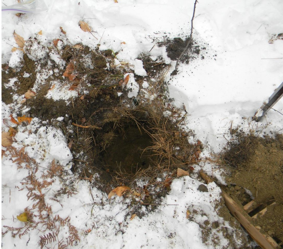
Figure 11. Photograph of Unit 3 (Z4-ST01-PS01). Excavation has been completed at 24 in. (60 cm) BS.
