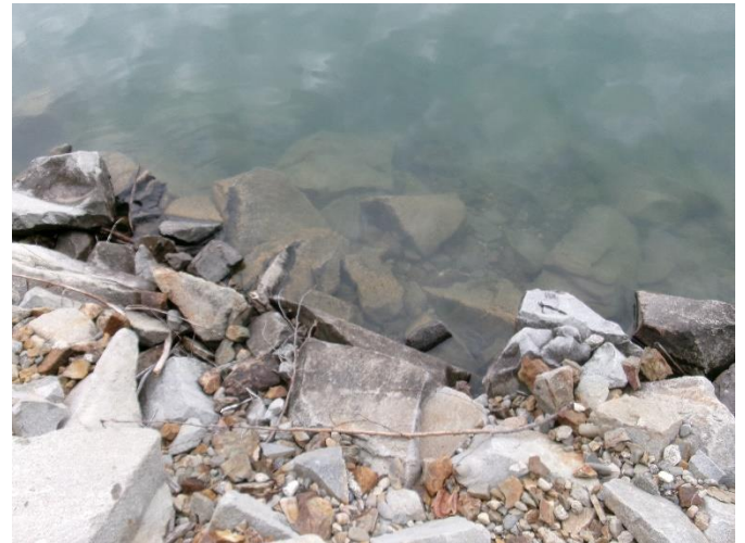
Representative photo of riprap along shoreline of project footprint during high water levels
