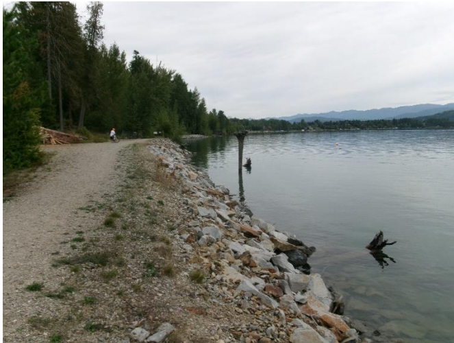
View of riprap shoreline along project footprint facing northeast
