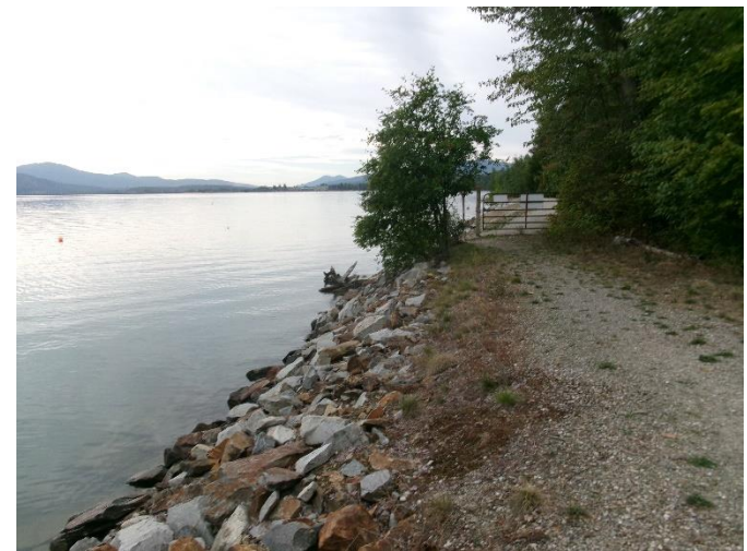
View of riprap shoreline along project footprint facing southwest
