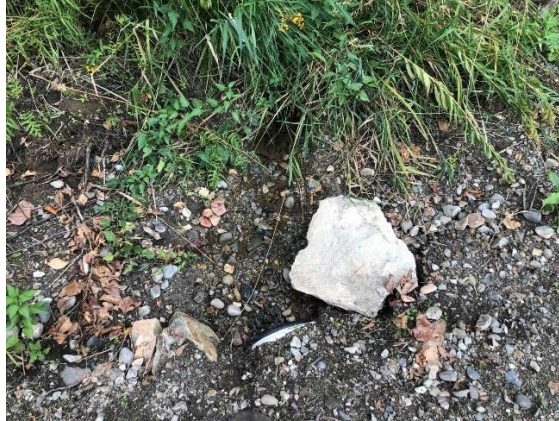
View of culvert inlet of Tributary A
