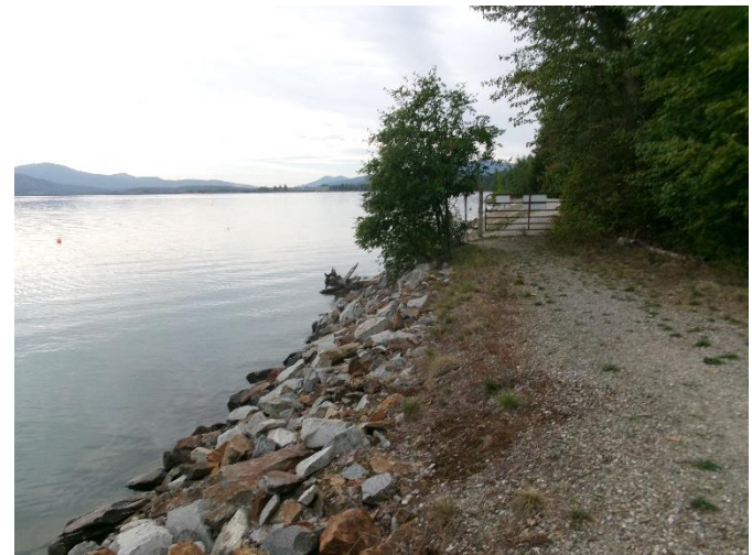
View of riprap shoreline along APE facing southwest
