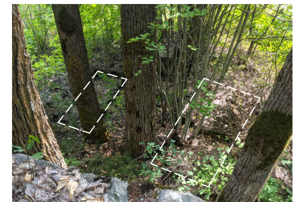
5.) CAREFULLY REMOVE VEGETATION GROWING ON AND AROUND EX. CONC STRUCTURES. REMOVE AS MUCH SOIL/MATERIAL AS POSSIBLE WITHOUT DISTURBING THE PHYSICAL STRUCTURES. POWER WASH CONC AFTER ALL EXCAVATION ACTIVITIES HAVE BEEN COMPLETED. SEE SHEET C5-B FOR EXCAVATION PLAN AND SHEET C6-B FOR GRADING PLAN.
