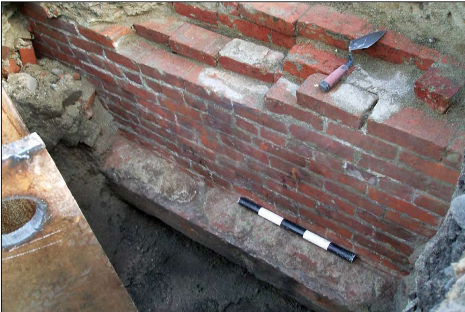
45KI1924, In WSDOT ROW for SR 99 Tunnel
