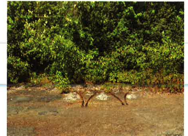
2.) PRESERVE AND PROTECT. CLEAN OUT AND EXCAVATE SOIL AROUND THE EXISTING SLAB AND METAL RAIL IN PREPARATION FOR NEW BLACK ROCK CONC SLAB. FORM CONCRETE AROUND EX. SLAB AND RAILROAD TRACKS. SEE SHEET C4
