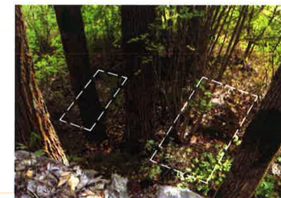
5.) CAREFULLY REMOVE VEGETATION GROWING ON AND AROUND EX. CONC STRUCTURES. REMOVE AS MUCH SOIL/MATERIAL AS POSSIBLE WITHOUT DISTURBING THE PHYSICAL STRUCTURES. POWER WASH CONC AFTER ALL EXCAVATION ACTIVITIES HAVE BEEN COMPLETED. SEE SHEET C5 FOR EXCAVATION PLAN AND SHEET C6 FOR GRADING PLAN.
