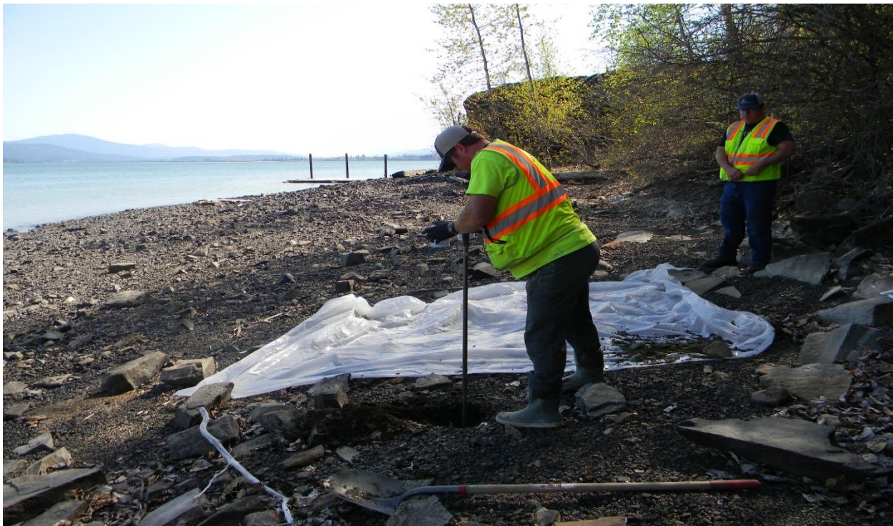
Figure 23. Photograph of SS-12 during excavation. The view is to the west.
