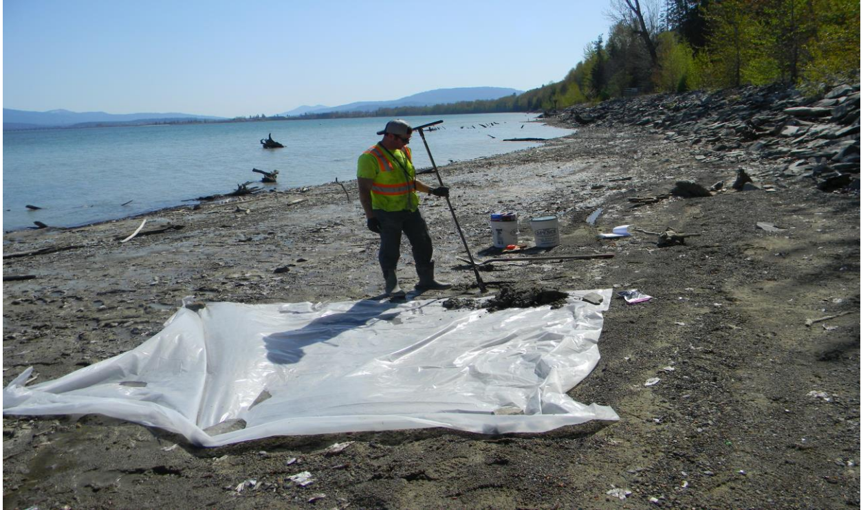
Figure 21. Photograph of SS-11 during excavation. The view is to the west.
