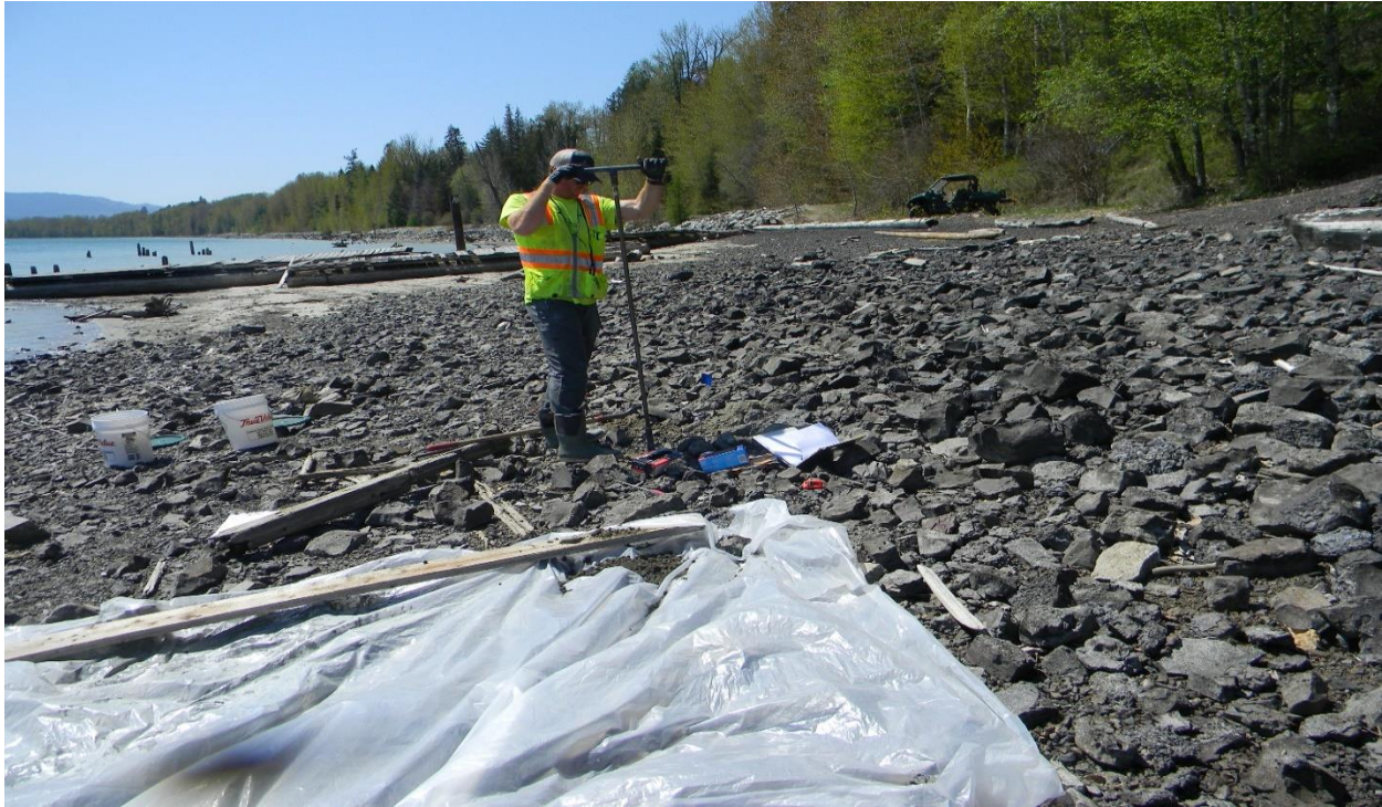
Figure 16. Photograph of SS-7 during excavation. The view is to the west.
