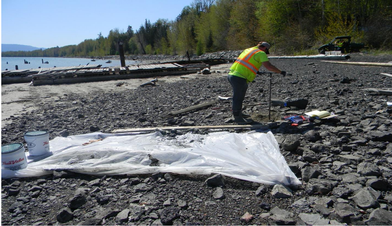
Figure 18. Photograph of SS-8 during excavation. The view is to the west.
