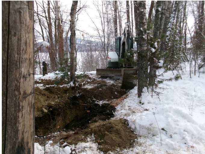
TP-1 backfilling facing southeast
