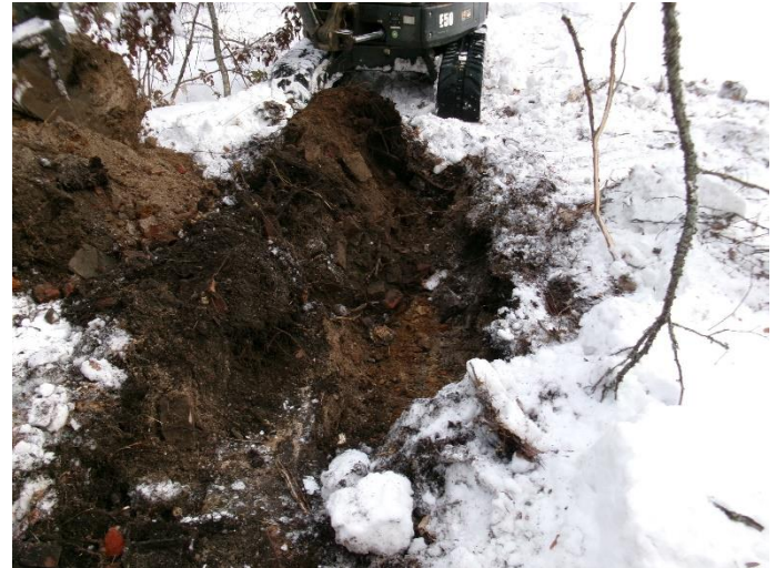
TP-2 moved test pit NE to avoid concrete footing
