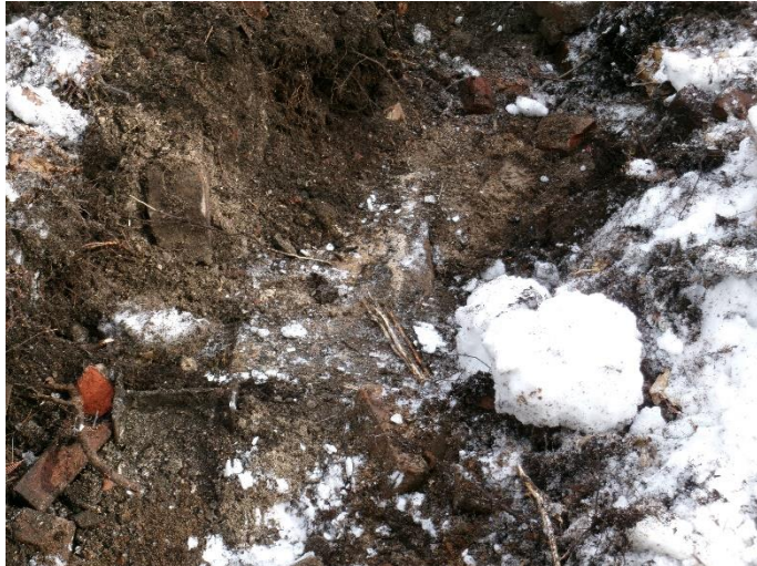
TP-2 concrete footing in top 0.5' of test pit
