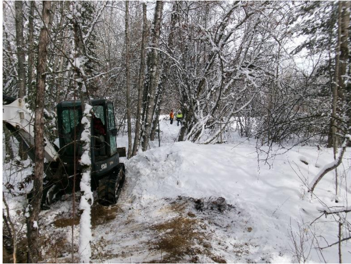
TP-2 backfilled facing northeast
