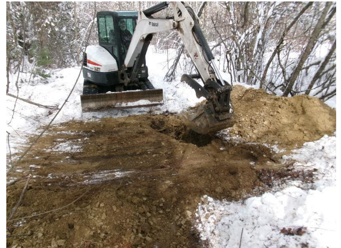
TP-3 backfilling facing north
