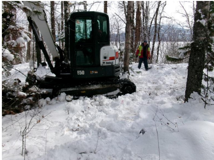
Excavating TP-1 facing east
