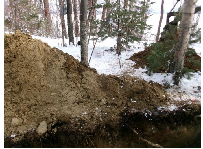
TP-1 spoils pile. 2-4' material on far right
