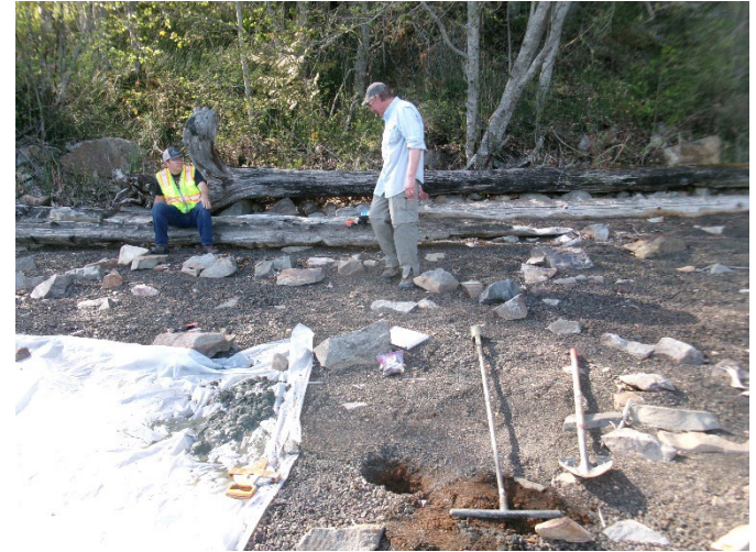
SS-13 soils and location facing north
