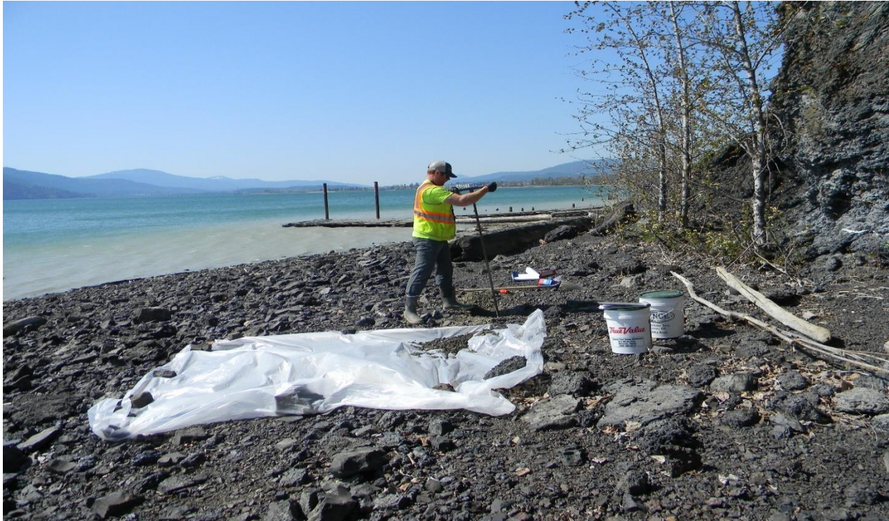
Figure 8. Photograph of SS-3 during excavation. The view is to the west.
