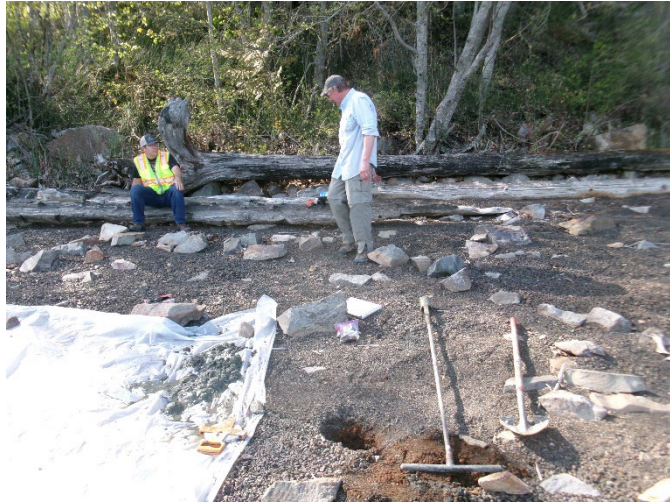
Equipment utilized for soil borings
