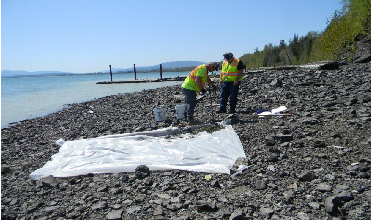
Figure 14. Photograph of SS-6 during excavation. The view is to the west.
