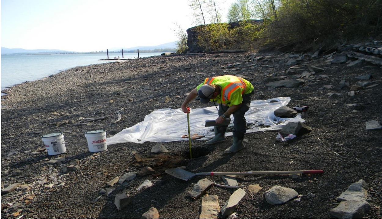
Figure 24. Photograph of SS-13 during excavation. The view is to the west.
