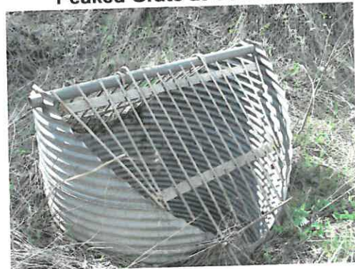
Peaked Grate at Culvert 38
