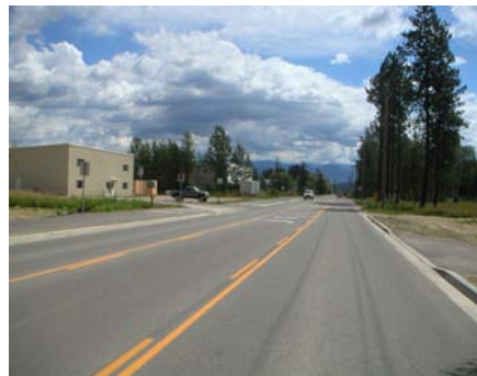
Kootenai Cut-Off Road provides a separated bikeway, a 2-way left-turn lane, and a drainage facility.
